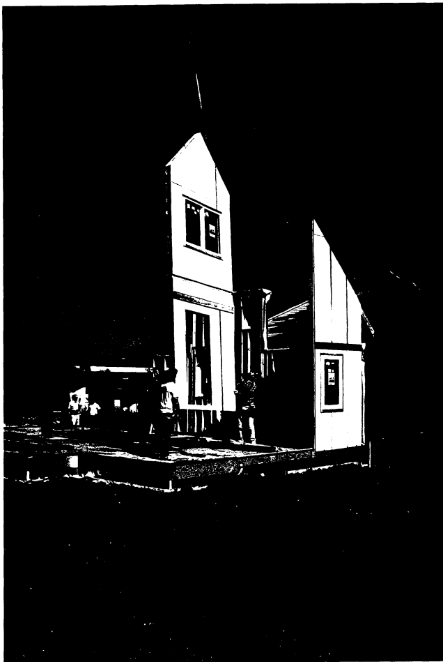
Fig. 3. 1-1/2 story prototype's open panels being craned into place. The exposed framing is visible in back walls.
