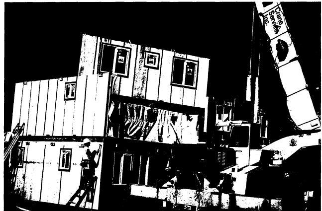
Fig. 5. 2 story prototype's closed panels being craned into place. The covering protecting the pre-installed gypsum board is visible at back walls.
